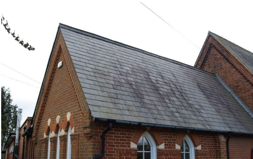
Slate tiles at Graveney Primary School.
