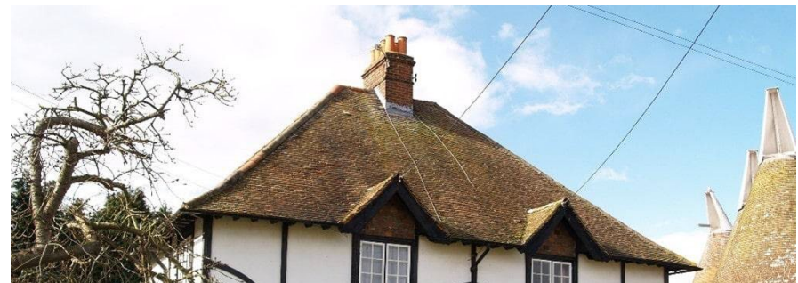
Tiles on roof of Poplar Hall Cottage.
