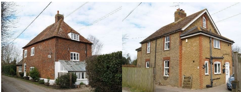
Brickwork of Oast House and Goodnestone Cottages.
