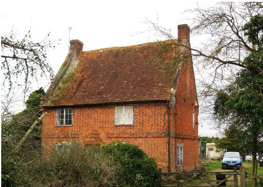
Brickwork to front of Murton's Farm.
