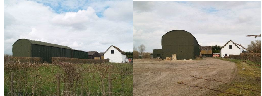
View towards Goodnestone Farm from footpath.
