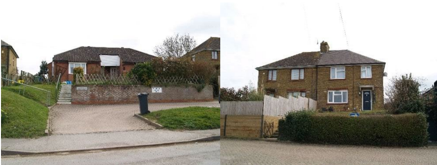
Housing further south of Harbour Cottages.
